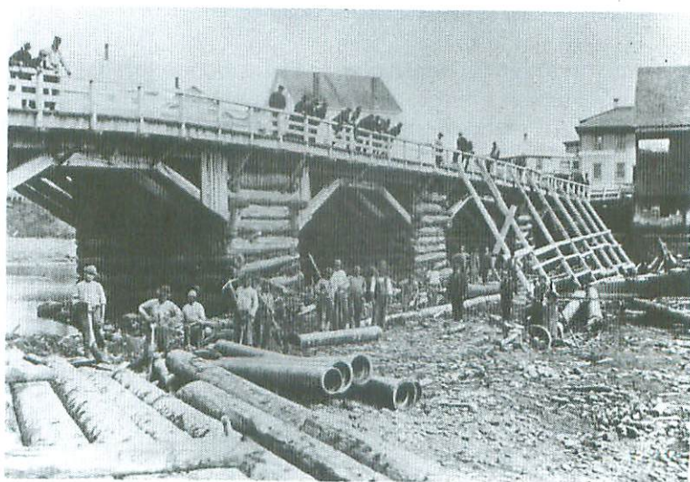
LAYING WATER MAIN ACROSS MEDUXNEKEAG RIVER AT UNION SQUARE 1885
